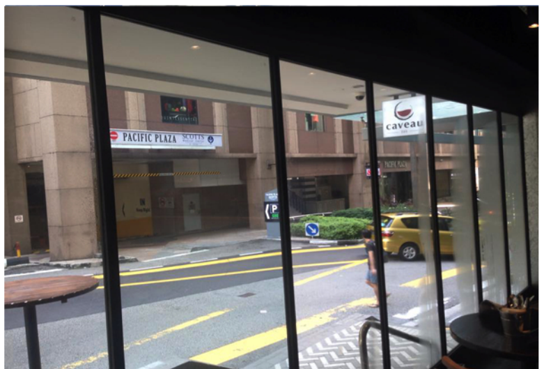
Caveau Wine Bar - First 2 Panels Installed
